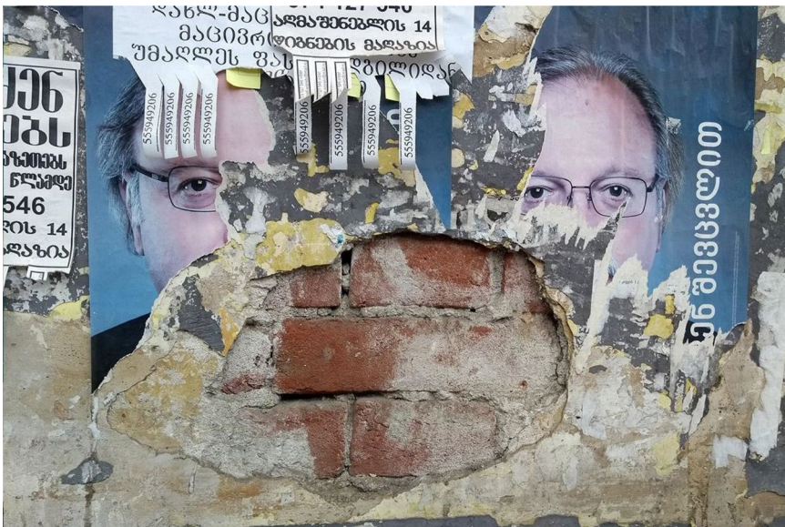
Figure 2. Street 'facade'- decaying posters, faces, adverts and phone numbers revealing hidden brickwork beneath the plaster. Nutsbidze Plateau II, Tbilisi (©2020 Photograph: Author).
